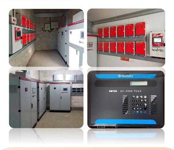
The chicken house control system is divided into two parts, the front-end electric control cabinet and the back-end strong current electric cabinet
